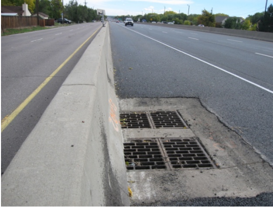
Looking east along 6 th Avenue
