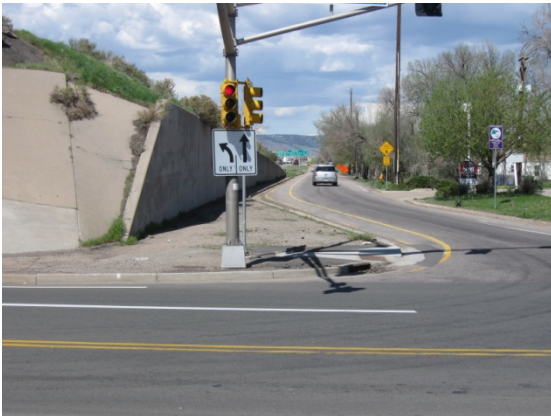
Looking west on north side of 6 th Avenue
