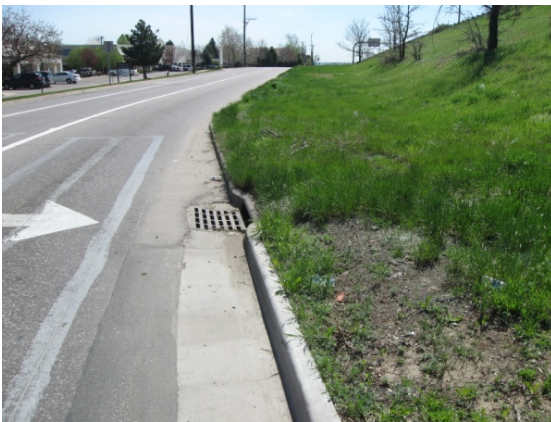
Looking east on north side of 6 th Avenue
