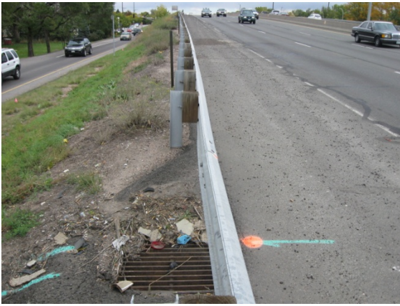
Inlet on 6 th Avenue, west of bridge
