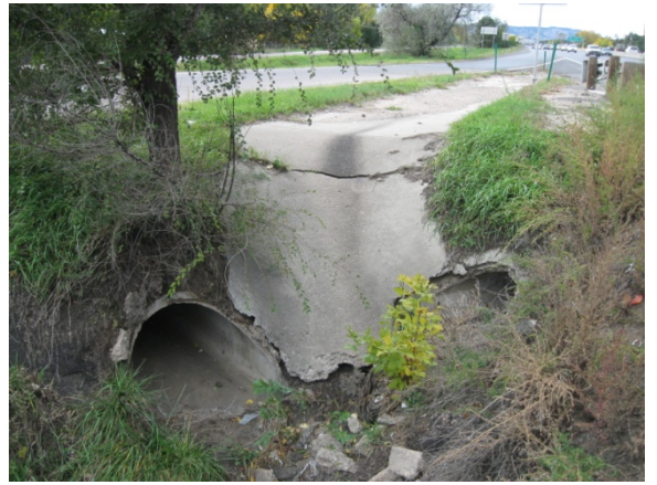
Spillway southwest of bridge, looking west
