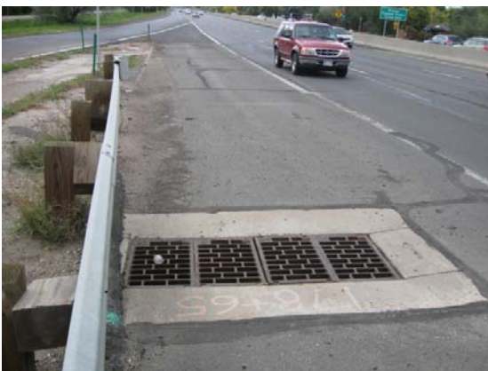
Inlet on 6 th Avenue, west of bridge
