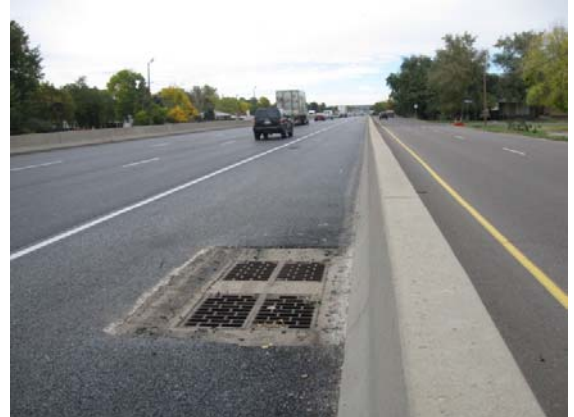
Looking east along 6 th Avenue
